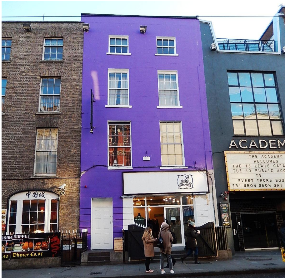
View of front elevation of 58 Abbey Street Middle.
