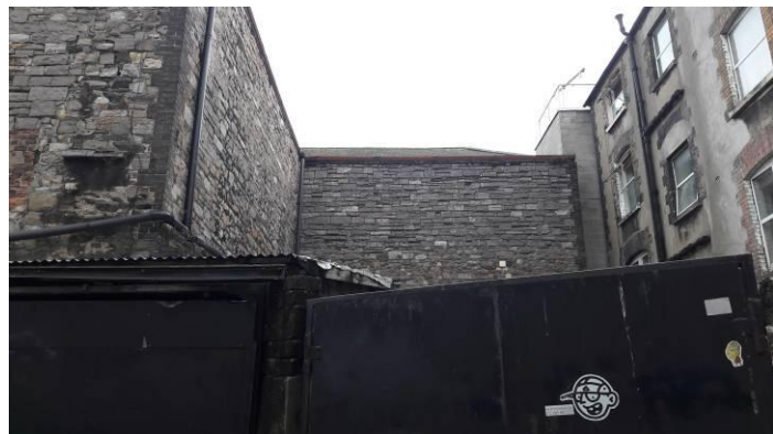
Side annex shed buildings
