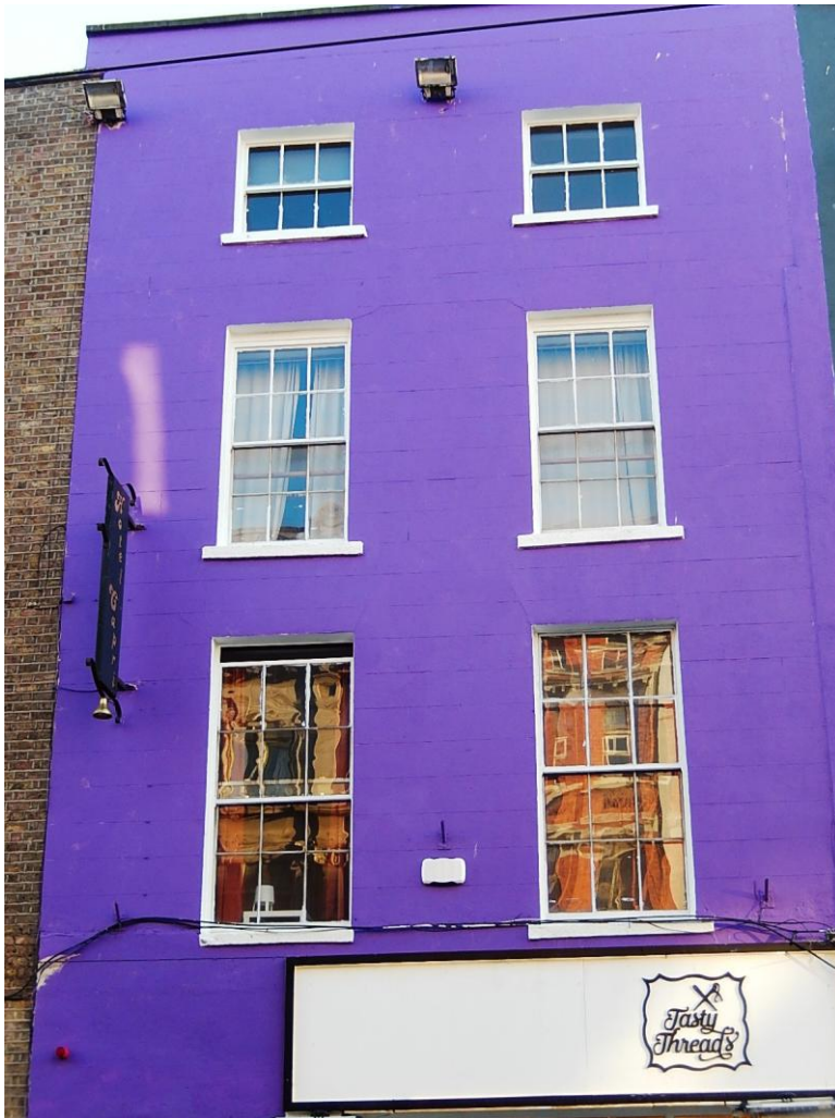
Upper floors to 58 Abbey Street middle with historic windows still intact.
