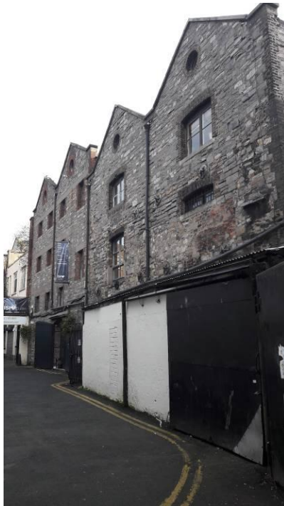
Front elevation of 4 Meeting House Lane with covered entrance steps to St Mary's Abbey
